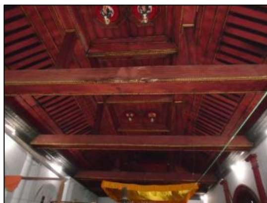
Figure 20. Timber Roof for Eastern Dormitory is Supported by Queen Post
