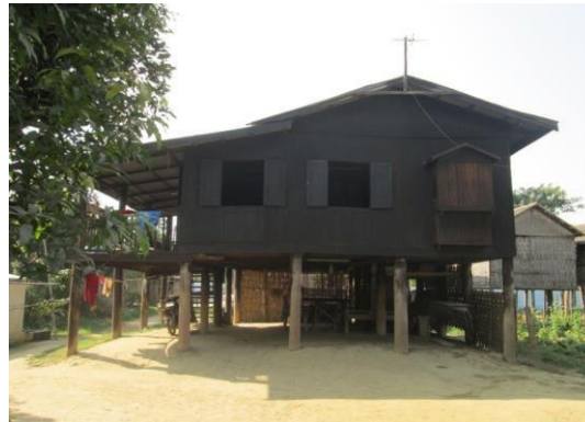
Fig (6) House Type (I) side elevation photo
