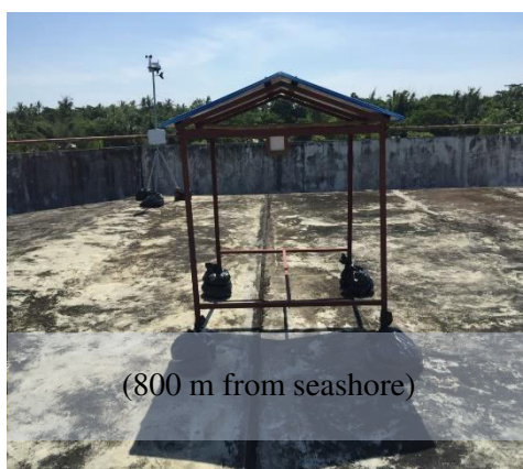
Figure. 3 Dry Gauze in the Sample House on the Roof Slab of Technical High School
