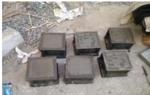
Fig.8 Casting of cubes
